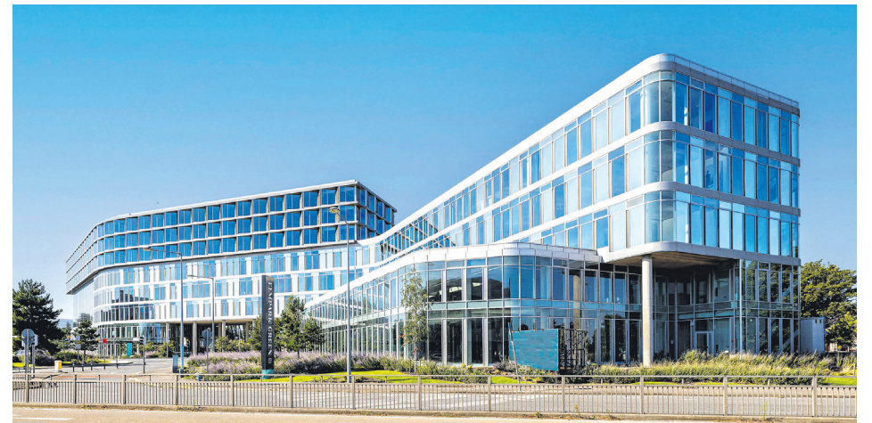
Elmpark Green: the entire scheme cost €550 million to build
