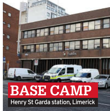
BASE CAMP Henry St Garda station, Limerick
